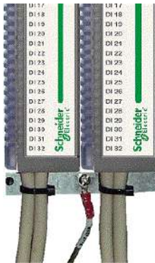
Figure 74 - Mounting cables to the cabinet or chassis
